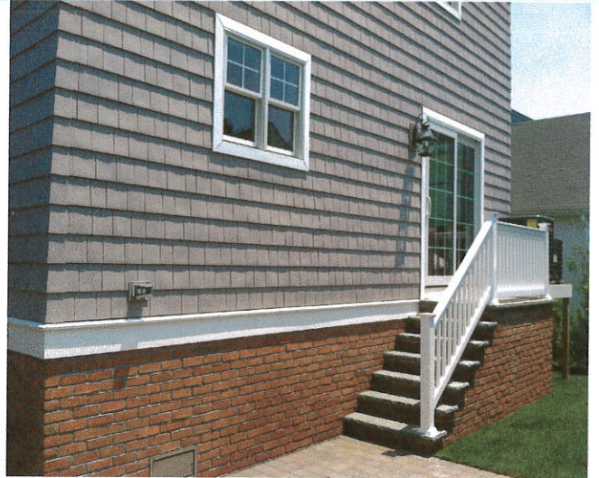
Rear View Date Taken: 07/02/2012
